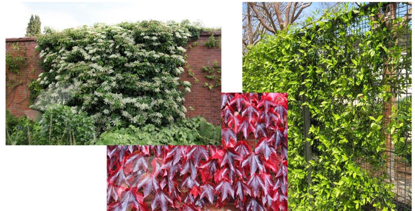
NORTH GREENROOF WALL AND HVAC SCREENING
